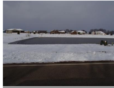
A new stormwater retention pond that is working in one of our subdivisions.....
