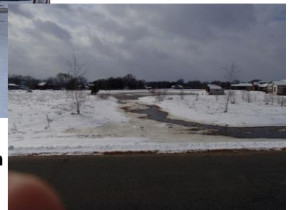
Drive with care in areas where water sometimes ponds on our roads during Spring thaws or during heavy rain events.
